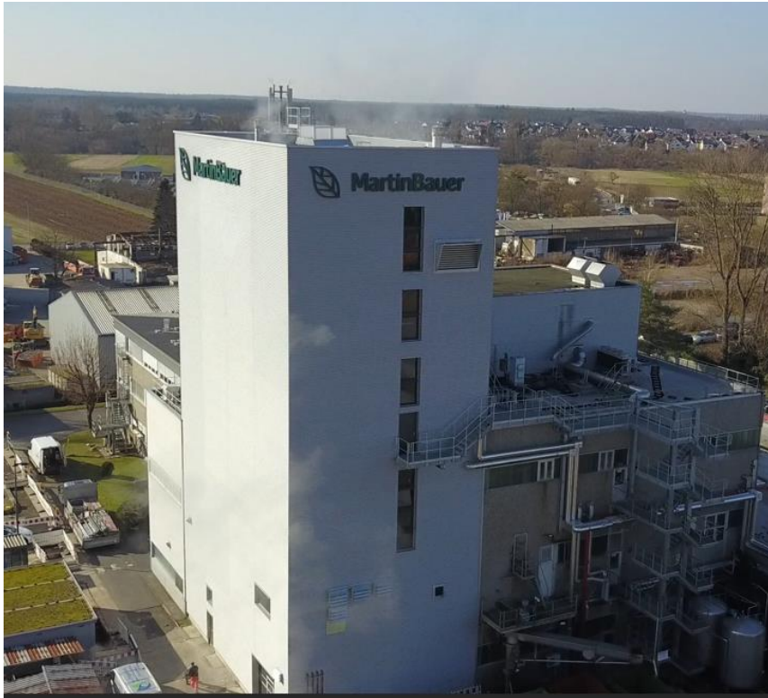
Figure 9 – New spray drying tower MartinBauer, Germany
