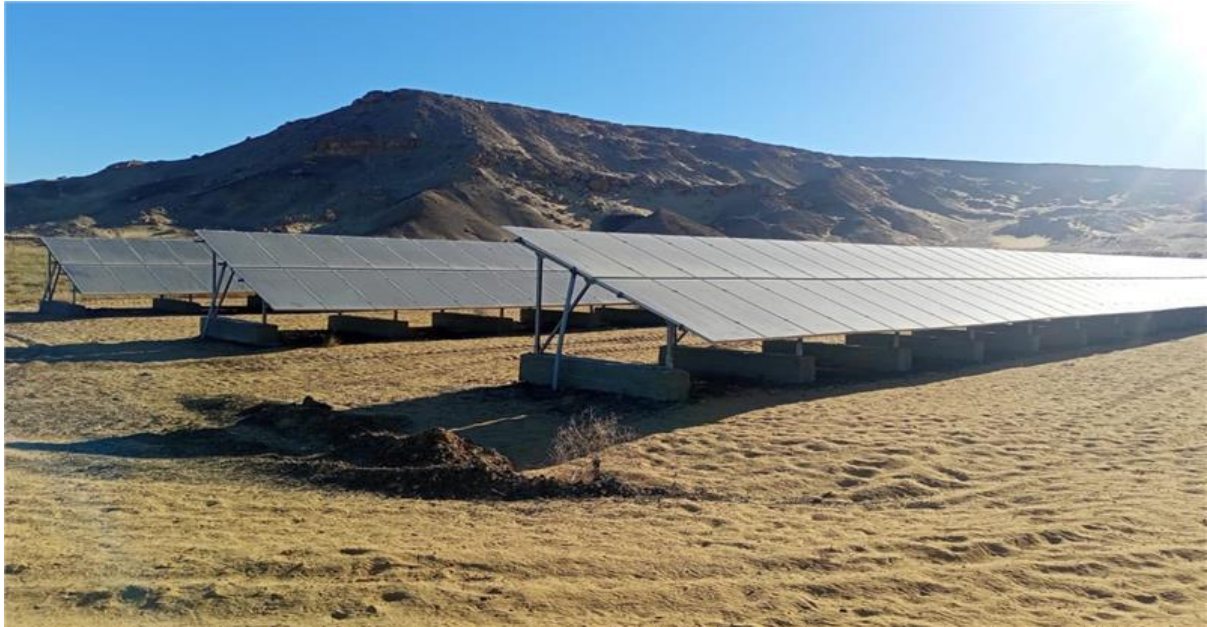
Figure 7 - Solar energy for efficient irrigation in Egypt
