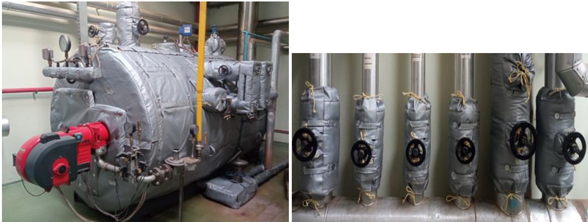
Figure 13 - Energy efficiency through insulation mats, MartinBauer, Germany
